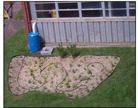
Connecting a soaker hose to your rain barrel is an efficient means of irrigation.
